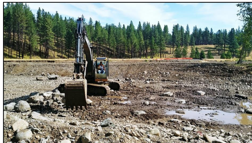
Constructing new channel riffle with imbedded boulders
