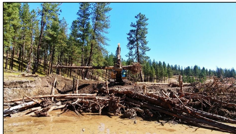
Constructing large wood jam structure
